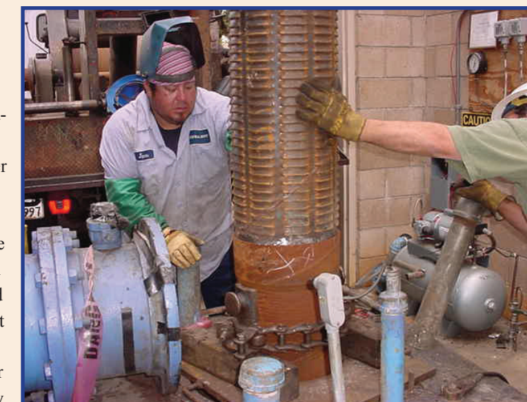
Well 22 being renovated to improve water quality and extend the life of the well.
