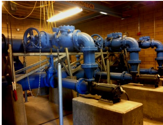
City of Guadalupe Water Pumping Station
