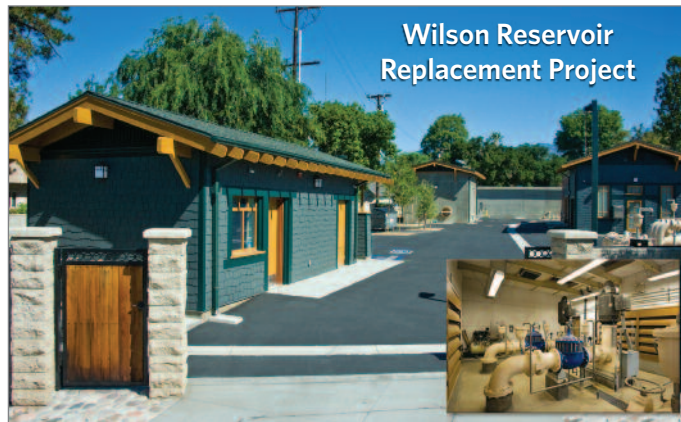
The century-old Wilson Reservoir was renovated this year. The old building was demolished and a new, reinforced concrete reservoir and pump station installed in its place. The new reservoir will hold 1.3 million gallons of water.
