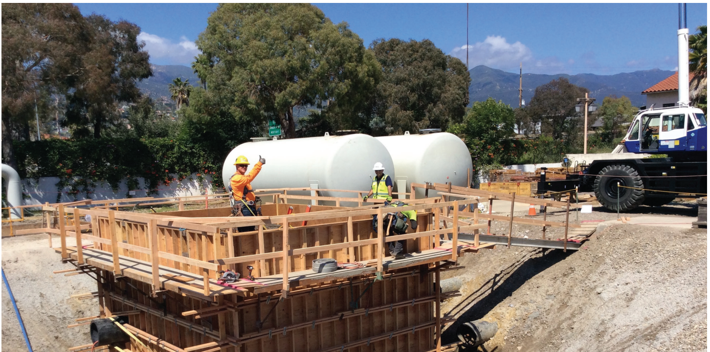
The Desal Plant is currently under construction.
